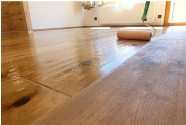
Fig. 2 Without a coating, UV light can interact with wood surfaces, causing discoloration and damage.
